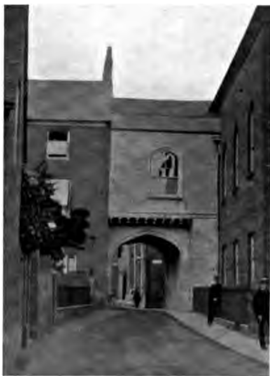
THE OUTER GATE.--BEFORE REBUILDING.
